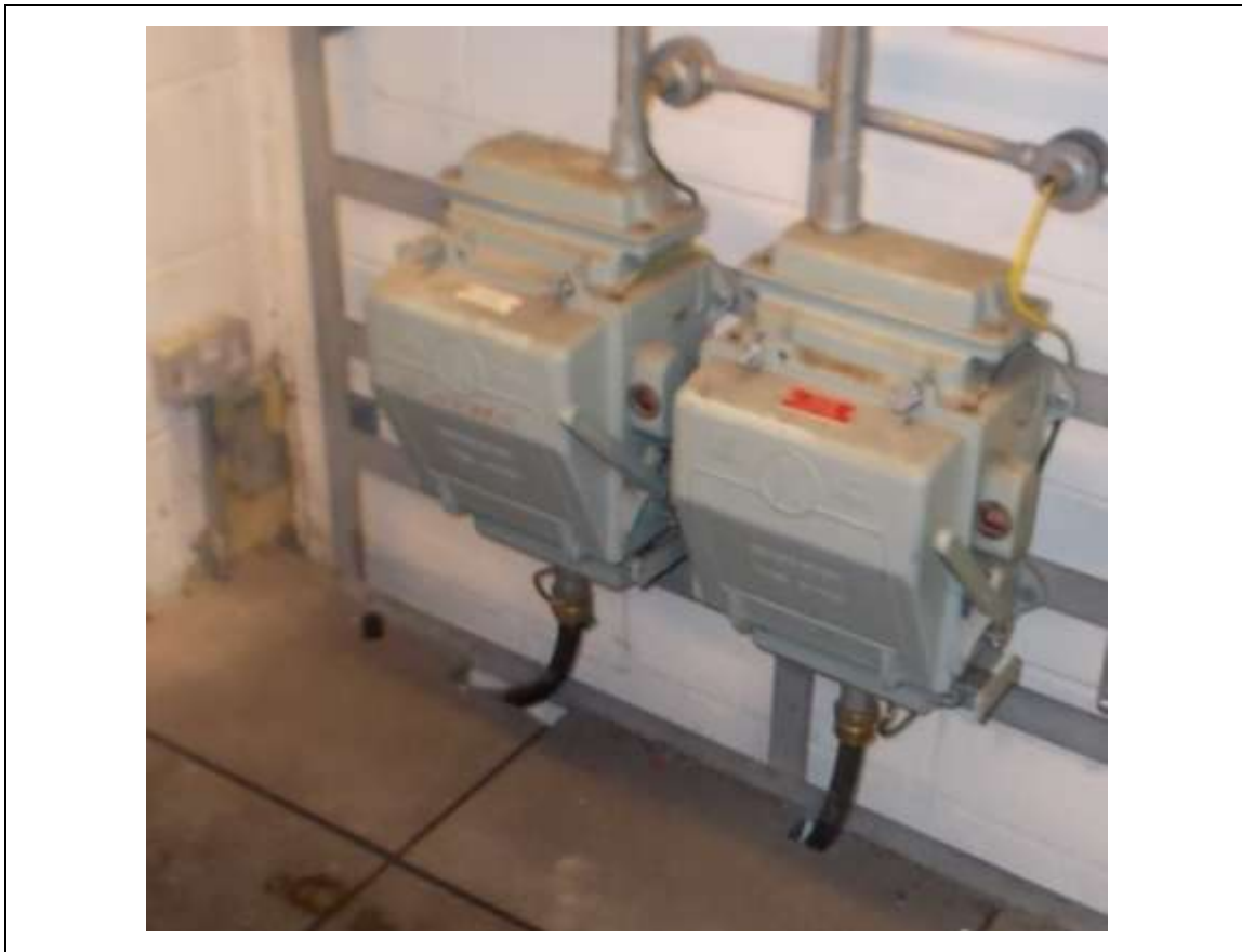
FIGURE 16: POSSIBLE ACMS WITHIN SWITCHGEAR IN CER, 3/731 - DESCRIPTION & RESULT OF ASSESSMENT (SAMPLE REF. P1(3))
