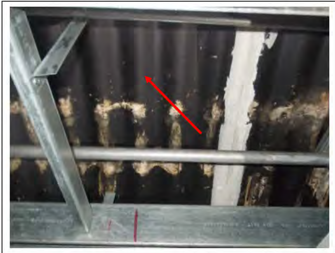
FIGURE 17: CONFIRMED ASBESTOS IN CELLACTITE IN OFFICE, 3/751 - DESCRIPTION & RESULT OF ASSESSMENT (SAMPLE REF. ECS 81505, ECS 81506, ECS 81507)
