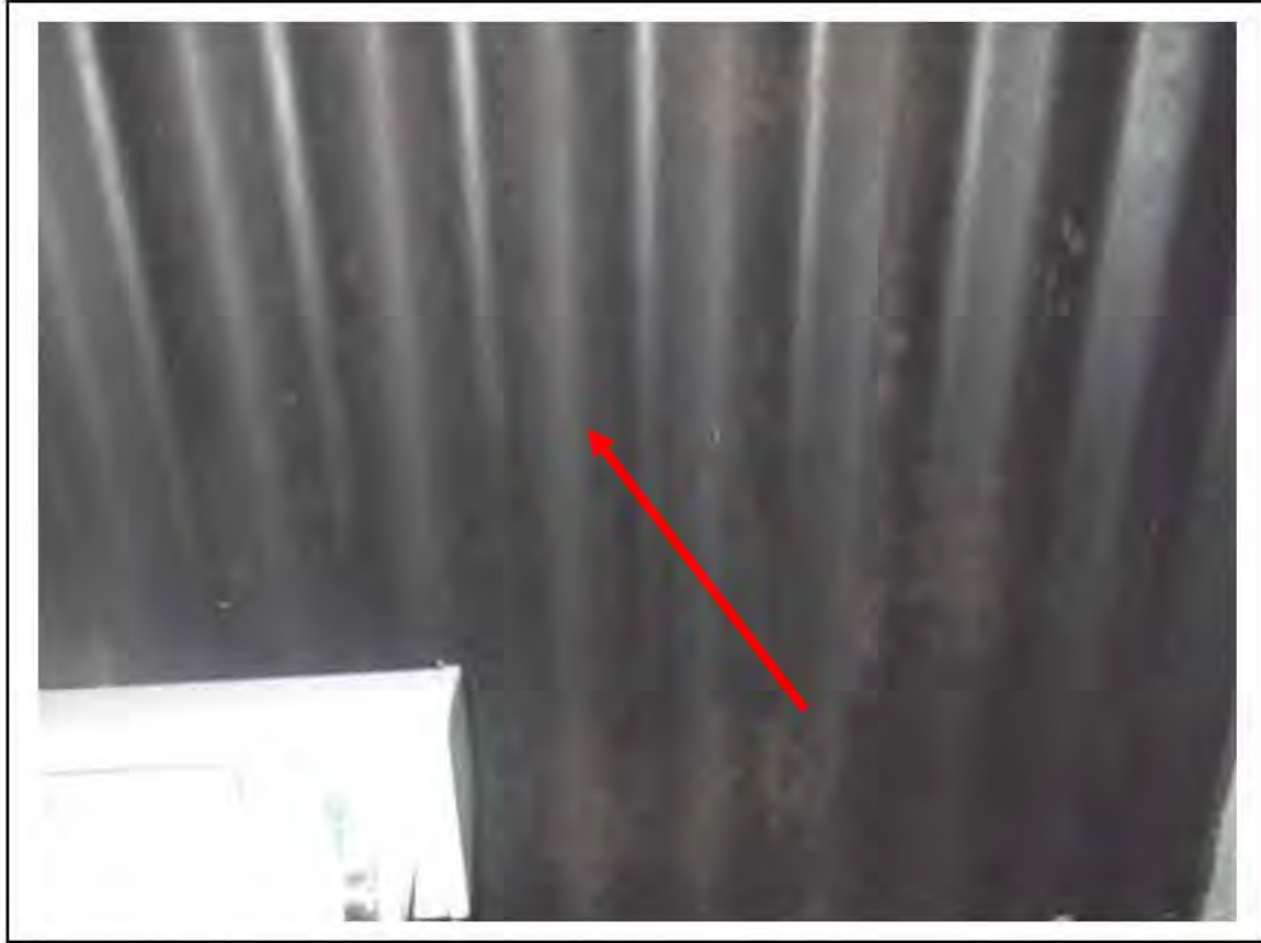
FIGURE 26: CONFIRMED ASBESTOS IN CELLACTITE IN LOBBY (PREVIOUSLY 6/236), 6/301 - DESCRIPTION & RESULT OF ASSESSMENT (SAMPLE REF. ECS 81579, ECS 81585)
