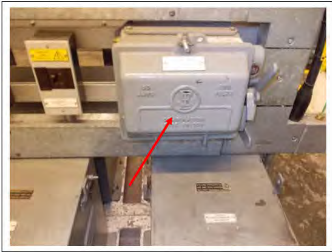
FIGURE 10: POSSIBLE ACMS WITHIN SWITCHGEAR IN CER, 2/746 - DESCRIPTION & RESULT OF ASSESSMENT (SAMPLE REF. P1(2))
